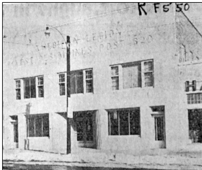
Figure 10: Newly finished 217 Fifth Street ( Des Moines Register , February 5, 1950)
