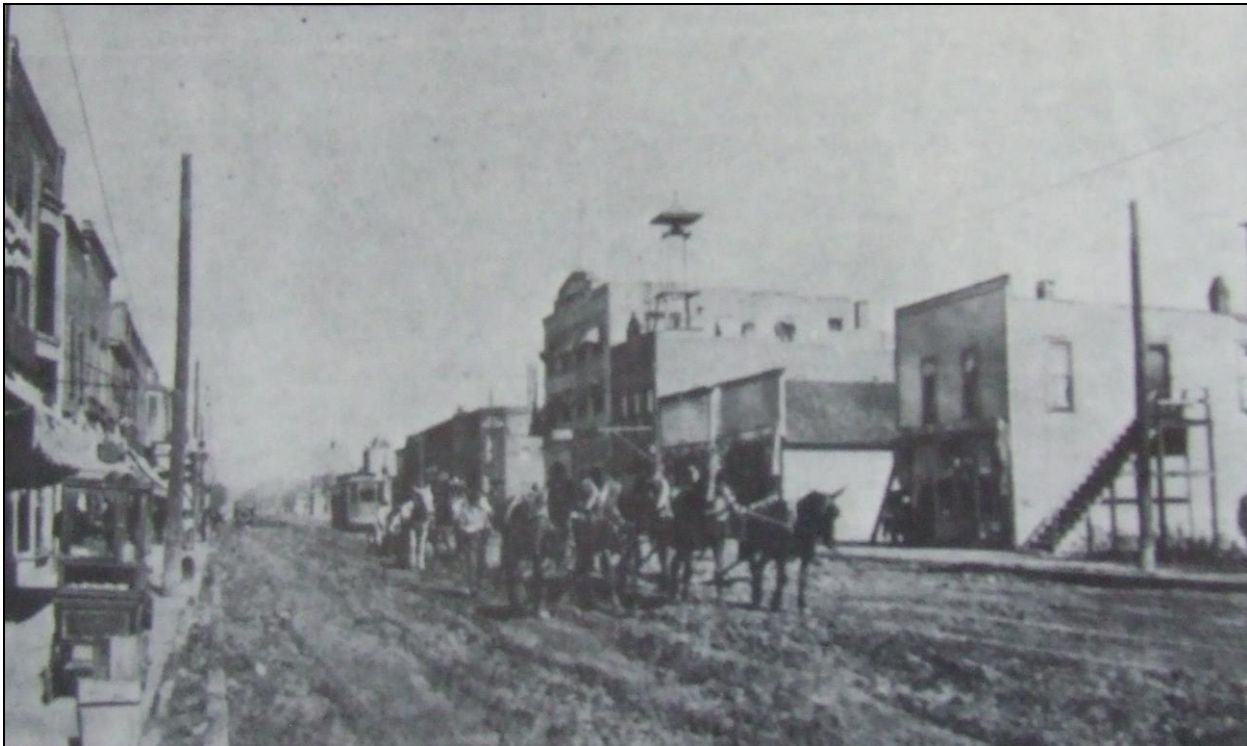
Figure 40: plowing lower Fifth Street preparatory to paving, looking northeast, 1915 (note no marquee on the Lyric Theater) (Jordan House Library and Archives)
