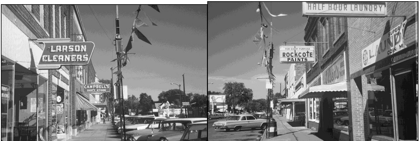
Figures 83-84: Blade sign example photos, October 1, 1964, 200 block Fifth Street looking north (Courtesy City of West Des Moines)
